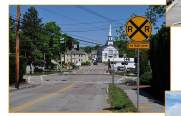
Commercial Street At-Grade Crossing in Braintree, MA with Flashing Lights and Four-Quadrant Gates
