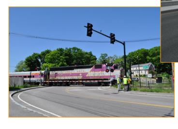
A Four-Quadrant At-Grade Crossing Intertied with a Traffic Signal in a Quiet Zone at South St., Hingham, MA
